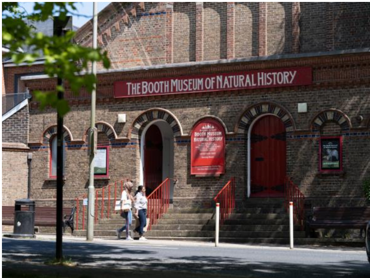
Fig. 1. Front facade of the Booth Museum, Brighton.
